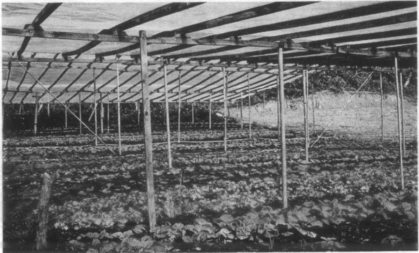
Fig. 8: Greenhouse on farm without ridge ventilation.
